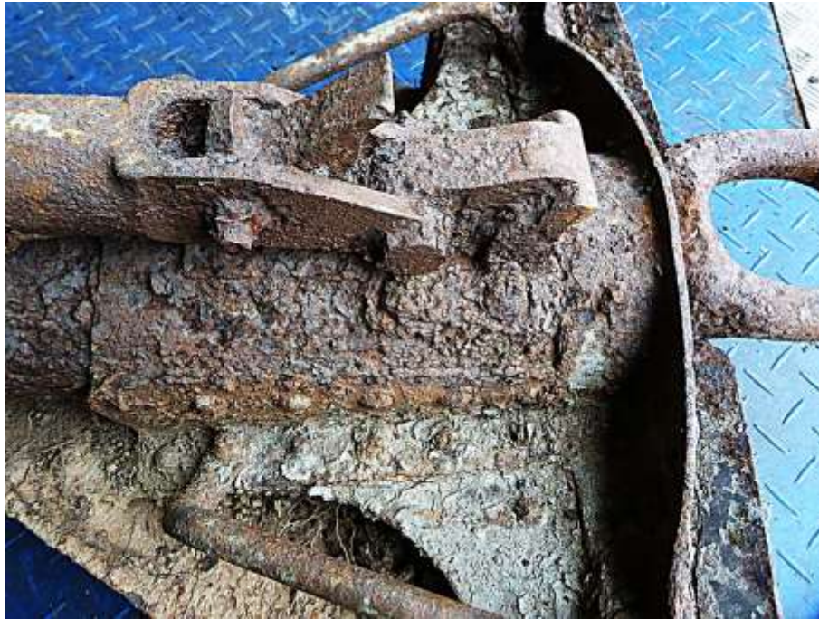
Figure 10 close up of the one of the lifting brackets mud and root visible
