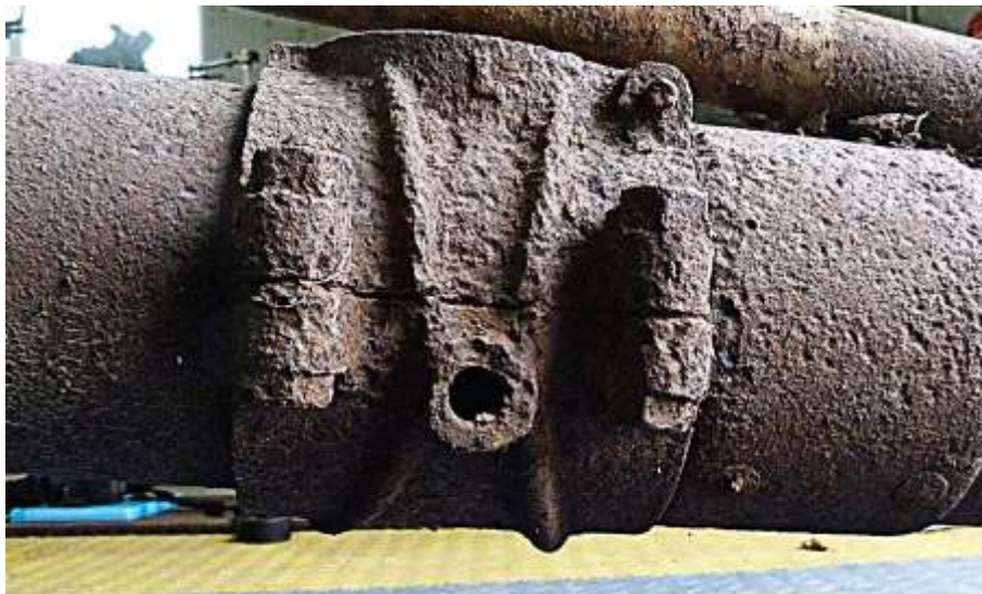
Figure 8 corroded part with damaged fastenings.
